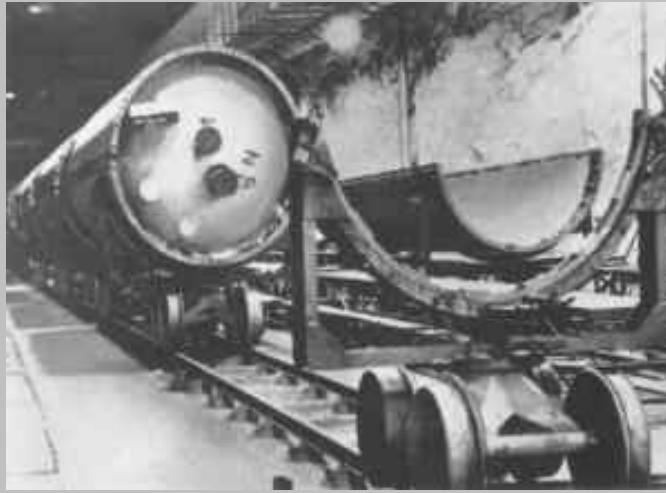
Part of the production-facilities in the B-Tunnel
